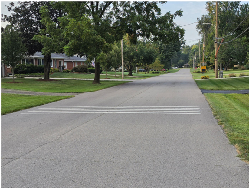
Ex. 4 – Rumble Strips & Speed Sign
